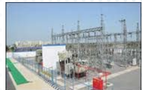
A view of the 66kV Rohini-28 grid substation.
