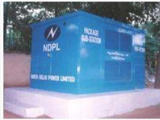
Packaged Substation
