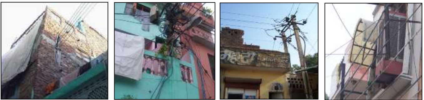
Fig 1: Public Apathy to Safety: Unauthorized Extension of Houses
