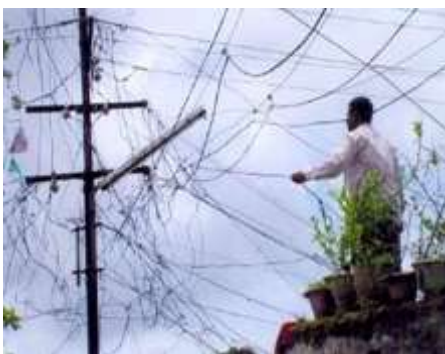
Snapshot of illegal hooking from the network
