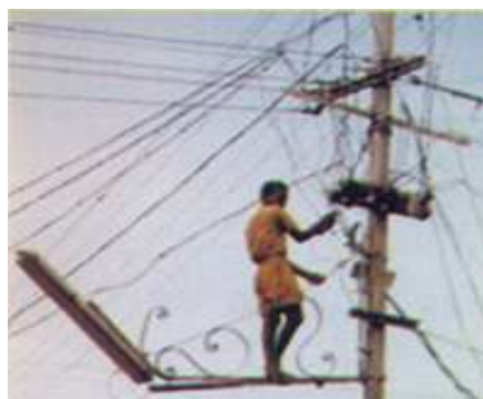
Snapshot of illegal hooking from the network
